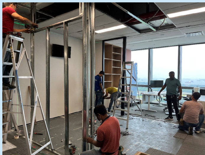
Construction of the new executive office
